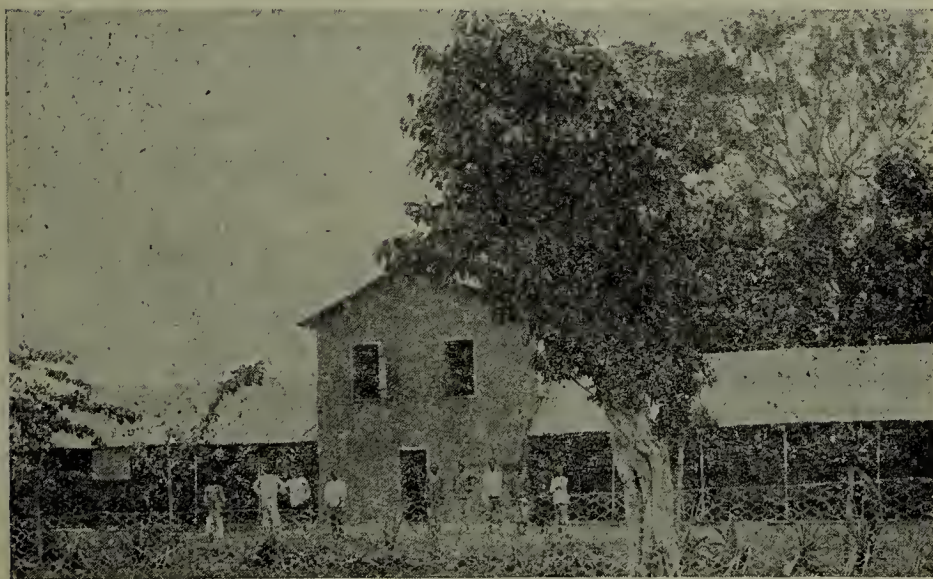
THEOLOGICAL TRAINING SCHOOL BUILDING, OGBOMOSHAW.
